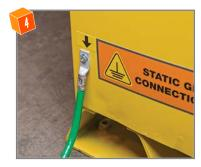
Ensure a full, metal-to-metal connection is established between the grounding fastener, grounding wire, and cabinet wall.
