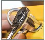
Using provided self-tapping, metal screws (B); attach the anchor plate (D) and D-ring (C) to bevel of the door by fastening screws into the pre-drilled holes. The straight length of the D-ring should sit and rotate freely under the raised portion of the anchor plate. (as pictured)
